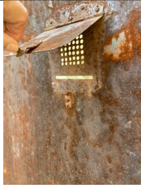
Peephole in the iron gate. Photos: Ivo Hammer 2021
