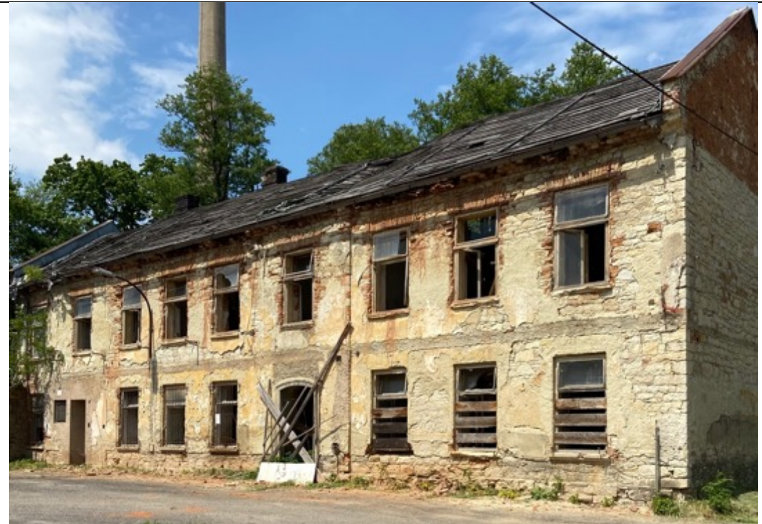
Former laboratory and workshop (SS-Bau des KZ Brnenec, German building). South facade. Profiled door frame with segmented lintel. Remnants of a tooth cut eaves.
