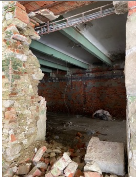
Schindler's Ark. View of the adjoining room to the east: ceiling made of double T-beams with vaulted spaces.
