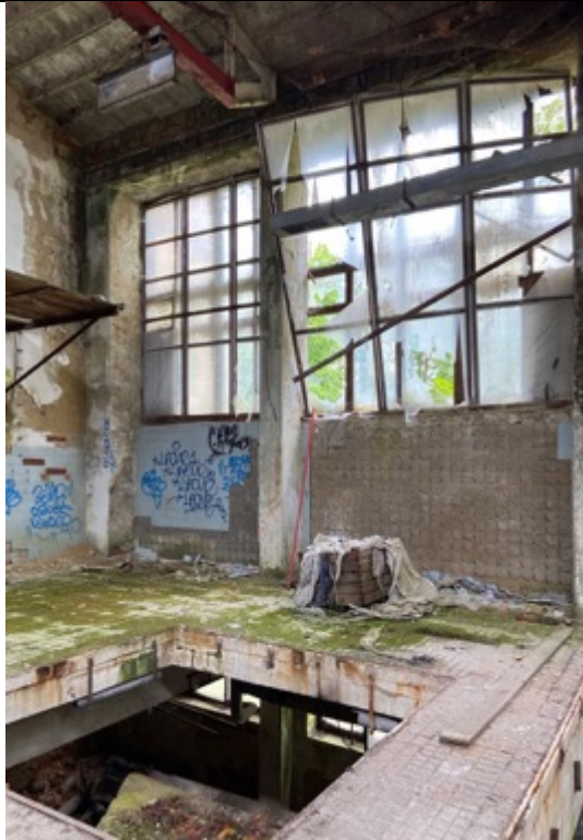
Schindler's Ark, dye works, northwest corner. Remnants of the crane
