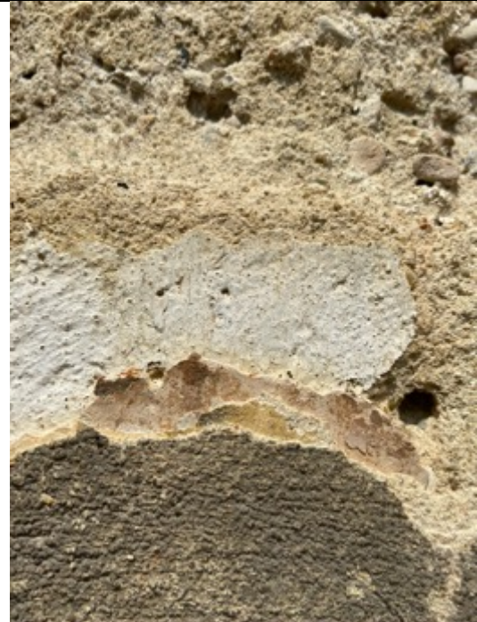
Fine plaster with the same mortar, only finer grain. Rubbed surface, very light yellowish-white, thin Freko whitewash. Approx. 5 whitewashes. Recent rub from (lime) mortar.
