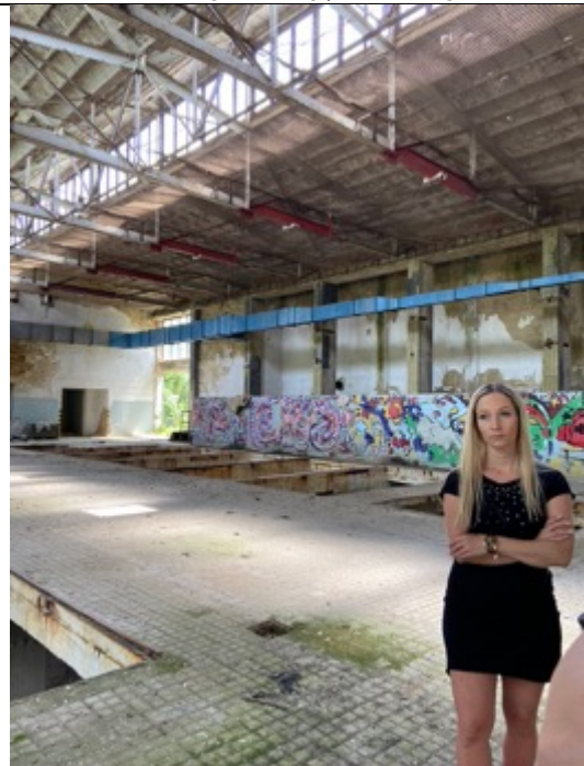
The walls are tiled up to the level of the sills of the north windows (blue, yellow, black). On the south side there is an additional tiled wall, probably as a splash guard (with recent wall paintings)
