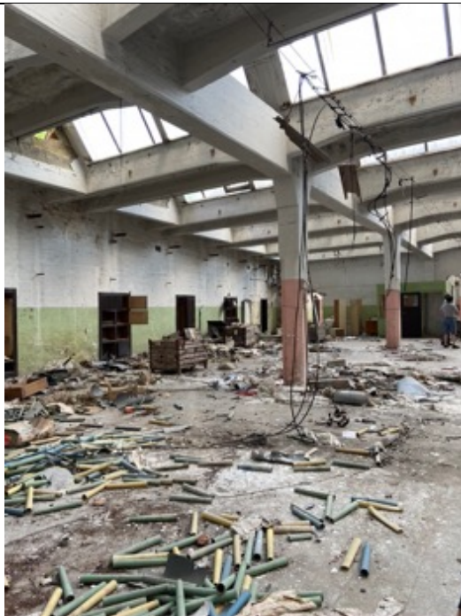
Spinning mill from approx. 1890, south interior, view to the northwest. Photo: Ivo Hammer 2021
