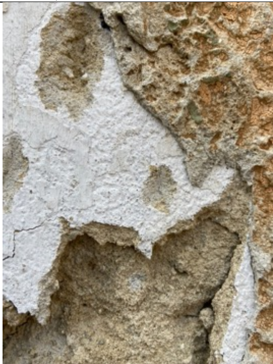
Residential building (management by Oskar and Emilie Schindler), facade detail: base plaster with yellowish-gray mortar with fine lime sparrows (dry slaking), fine plaster with the same mortar, only finer grain size.
