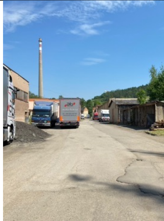
Northern part of the factory, looking north; in the background the former laboratory (SS building) and Schindler's Ark. Photo: Ivo Hammer 2021
