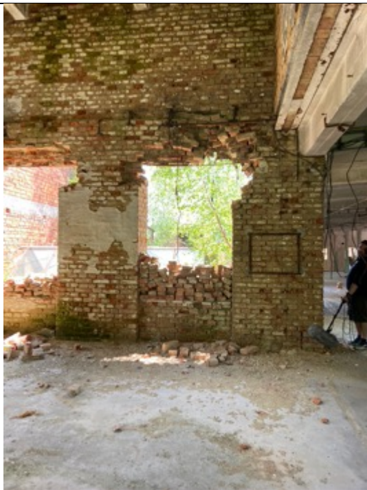
Schindler's Ark, 2nd floor, reinforced concrete hall, northern annex room, view to the south. Photo: Ivo Hammer 2021
