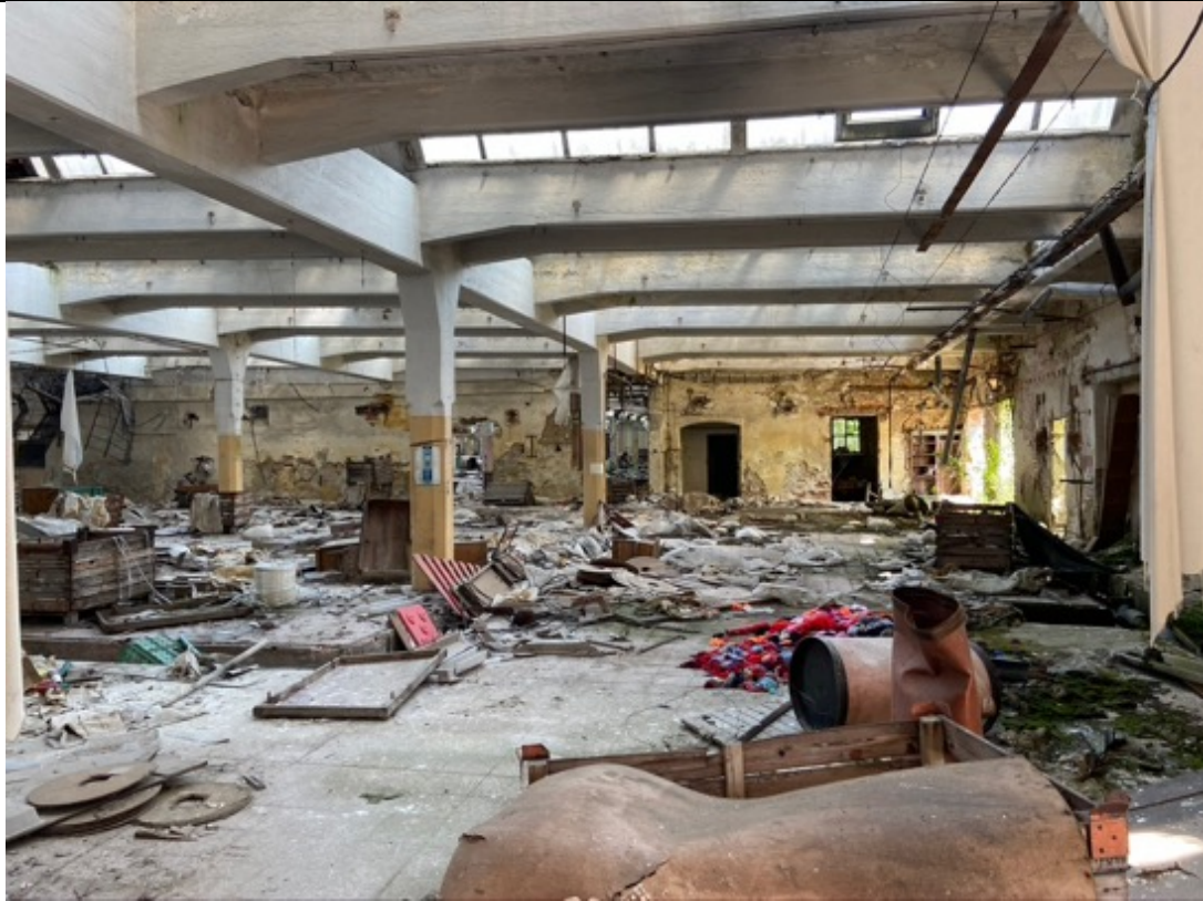
Spinning mill from approx. 1890, south interior, view to the north.
