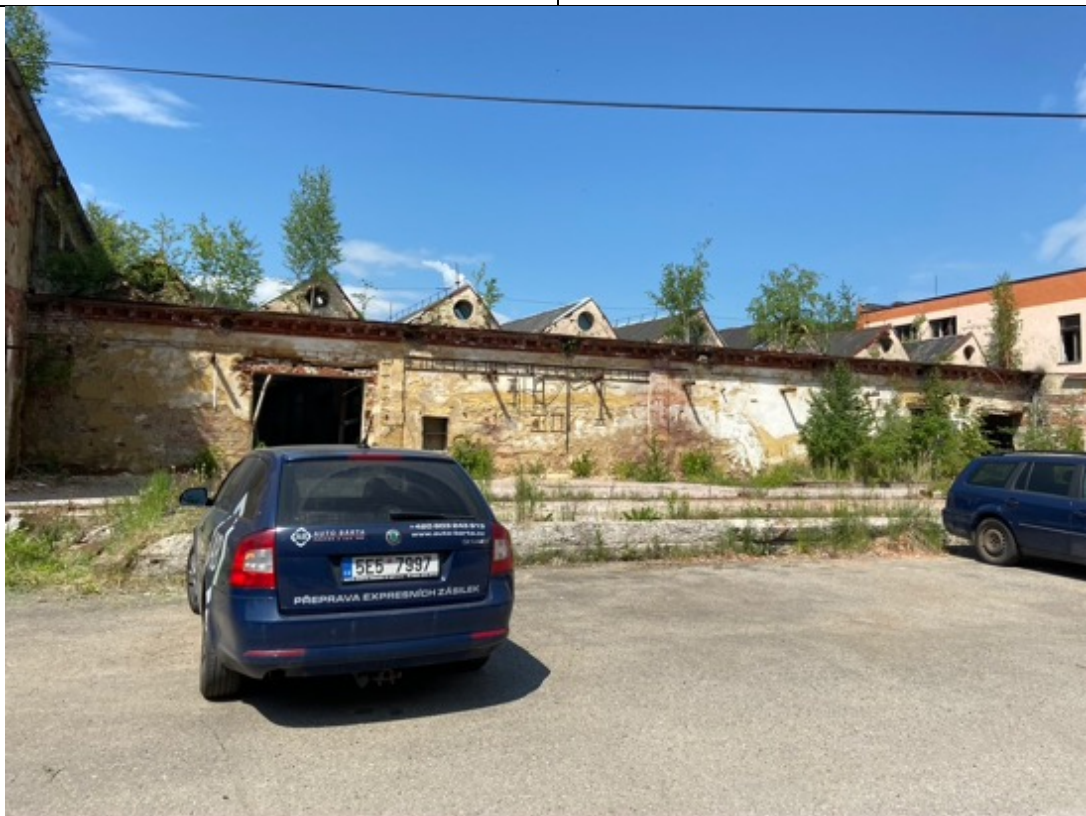
Spinning mill from approx. 1890, outer facade of the southernmost part, the later) vestibule has been removed; Structure of the smooth plastered façade with pilaster strips and serrated eaves made of brick, originally presumably yellowish-white lime paint, later several whitewashes in yellow and pink. The oculi of the hypetheral roof are bordered with fascia. The eaves of the roof gable may have originally only been protected with sheet metal. Photo: Ivo Hammer 2021
