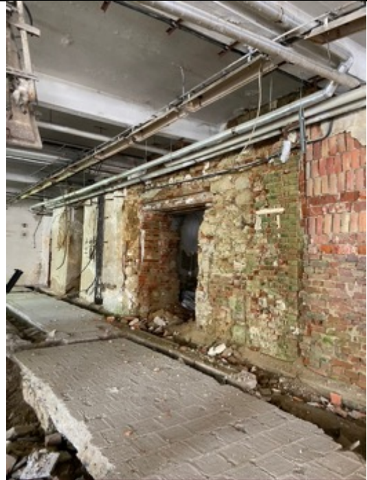
Schindler's Ark, ground floor, reinforced concrete hall, view to the northeast. Breakthrough through stone and brick wall. Bricking up a window. Photos: Ivo Hammer 2021
