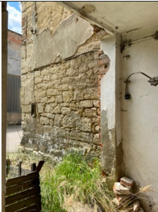
Schindler's Ark, east wall, detail of the south-east corner: stone masonry, sloping base
