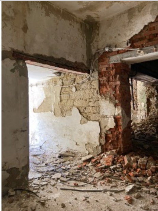
Conversions in the area of the annex building Photos: Ivo Hammer 2021
