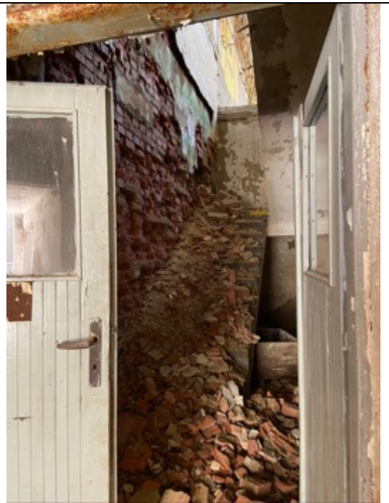
Space between Schindler's Ark and the annex to the dye works: concrete stairs. Photos: Ivo Hammer 2021
