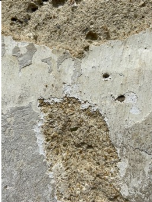
Former laboratory and workshop (SS-Bau des KZ Brnenec, German building). Details of the south facade (lower edge of the picture approx. 10 cm). Base plaster with yellowish-gray mortar with fine lime sparrows (dry slaking),
